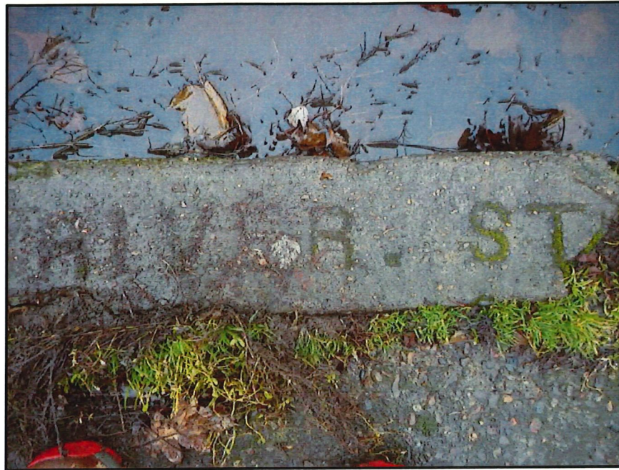
Figure 57. SNS 1, located at the southwestern corner of the intersection of E Sixth and S River Streets.
