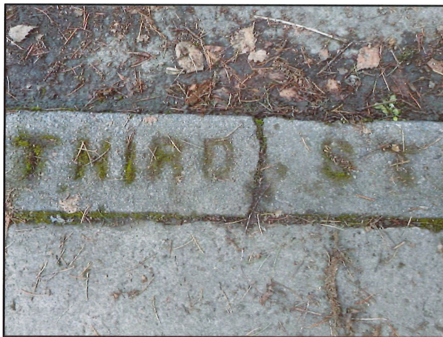
Figure 56. SNS 13, located at the southeastern corner of the intersection of E Third and S Chehalem Streets.
