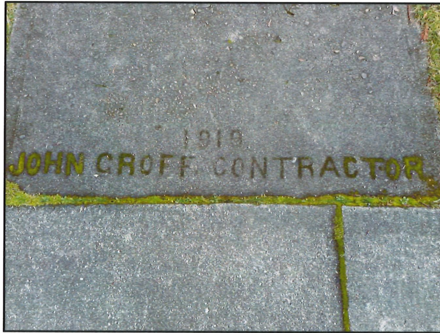
Figure 34. PS 19, located at the corner of SW corner E Sherman and N Washington St.
