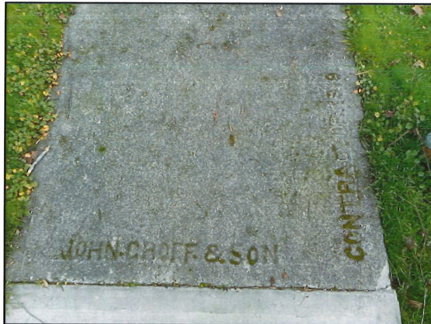
Figure 35. PS 21 located on the southern side of E Fourth Street, between S Meridian and S Center Streets.
