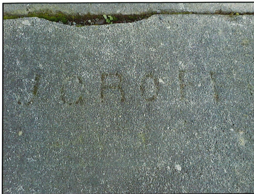
Figure 36. PS 23, located on the W side of N Garfield St., above E First Street.
