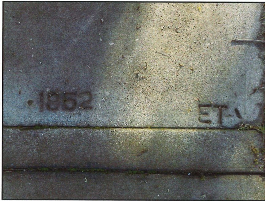
Figure 42. PS 2, located at the southeastern corner of the intersection of E Fifth and S School Streets.
