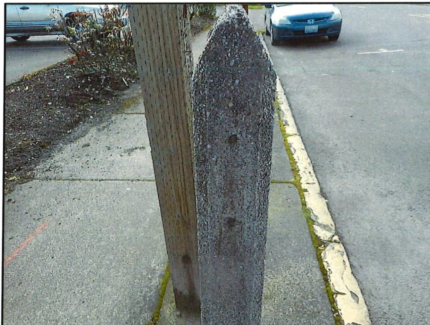
Figure 27. Close up of missing mailbox attachment on MP 5, located at the intersection of E First and S Main Streets.
