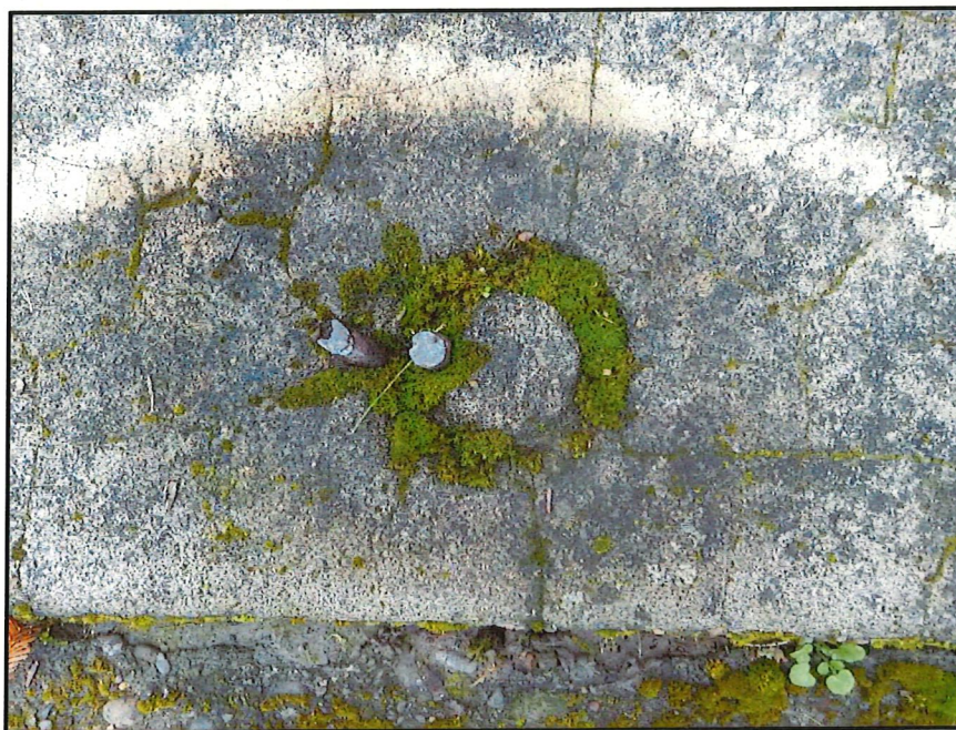
Figure 13. The remnants of HR 7, located at the intersection of E Sheridan and N Blaine Streets.
