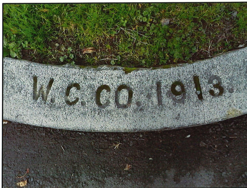
Figure 39. PS 8, the most legible of this group of stamps attributed to the Warren Construction Company, located at the northwestern corner of the intersection of E Fourth Street and S Main Street.
