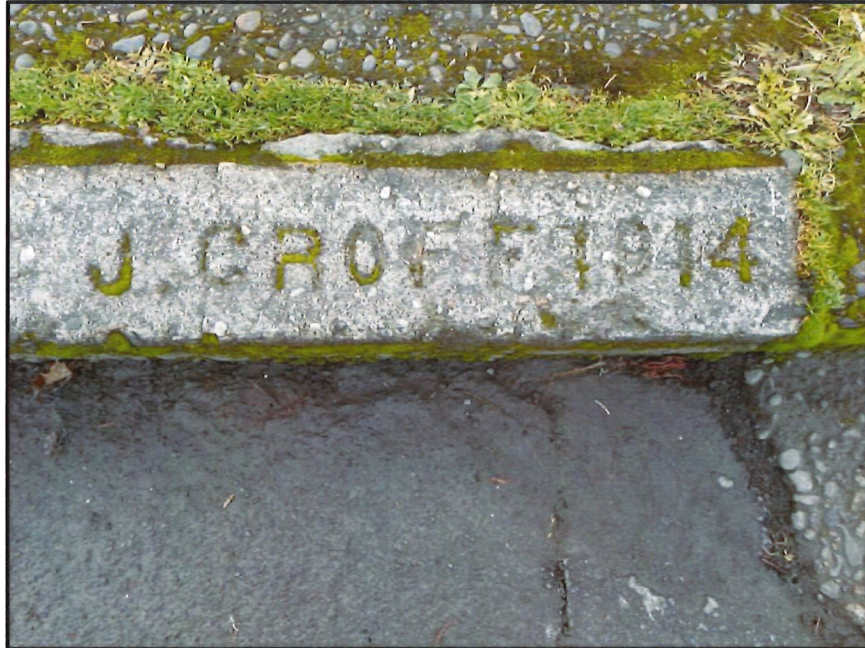
Figure 31. PS 6, located at the northeastern corner of the intersection of E Fifth Street and S Dayton Avenue, as described in Ordinance 344 (1914).
