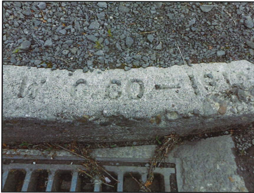
Figure 40. PS 15, at the northwestern corner of the intersection of E Sheridan and N College Streets.
