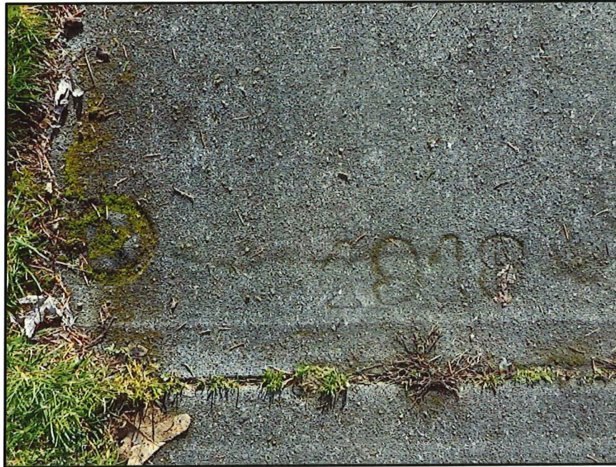
Figure 52. R 1, located on the east side of S Howard Street, between E Fourth and E Fifth Streets.
