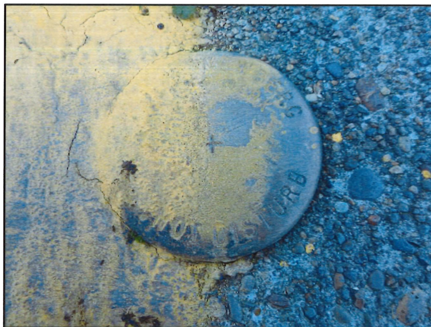
Figure 88. Benchmark 2, located at the southeastern corner of the intersection of E Third and S Edwards Streets.
